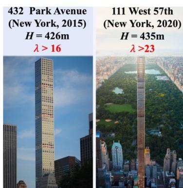
Fig. 1 High-rise buildings with super large aspect ratio
